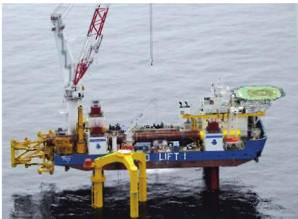
Plate 7 Figure 11.55 Tripile structure after installation. The yellow pile tops, which sport circumferential stripe markings, extend up to platform level with the cylinders above forming part of the three-arm transition structure. Reproduced by permission of BARD Group/Scheer
