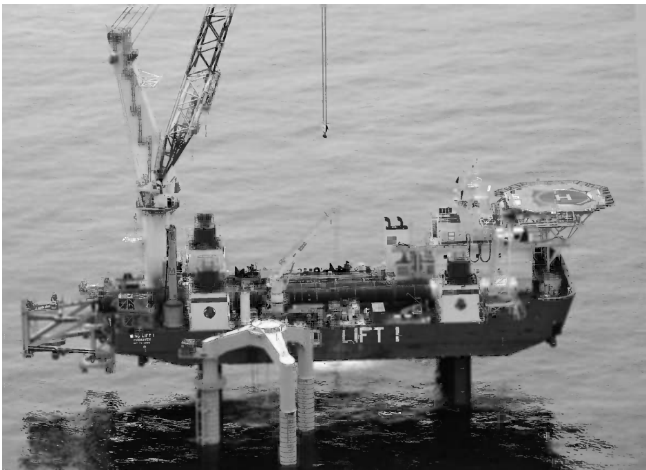
Figure 11.55 Tripile structure after installation. The yellow pile tops, which sport circumferential stripe markings, extend up to platform level with the cylinders above forming part of the three-arm transition structure. Reproduced by permission of BARD Group/Scheer. See Plate 7 for the colour figure
