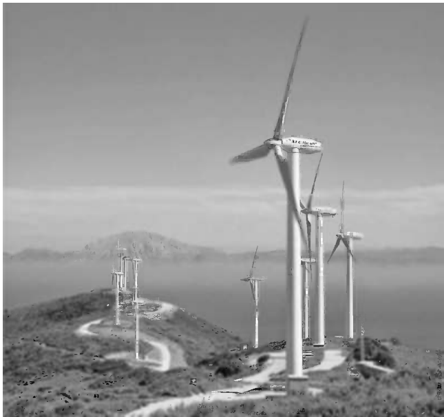
Figure 9.4 Wind farm of 600 kW turbines, Tarifa, Spain. Reproduced by permission of NEG MICON
