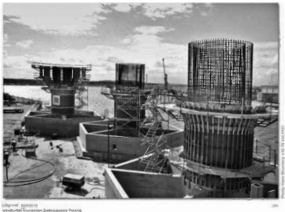
Figure 11.48 Gravity bases for Lillgrund under construction on barge at quayside at Swinoujscie. (Lillgrund Pilot Project, 2008). Reproduced by permission of Vattenfall. See Plate 4 for the colour figure
