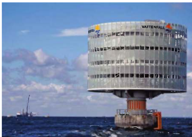
Plate 8 Figure 11.59 Offshore sub-station at Lillgrund. Lillgrund Pilot Project, 2008. Reproduced by permission of Vattenfall
