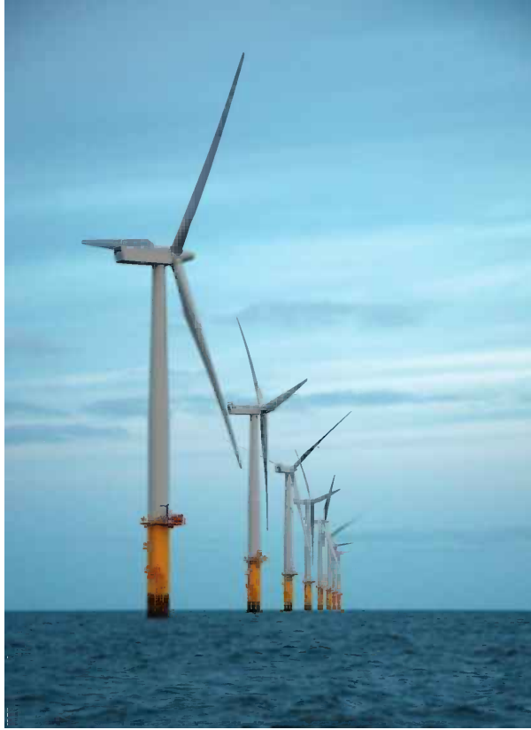
Plate 1 Figure 1.2(a) Rhyll Flats Offshore Wind Farm: 25 \times 3.6 MW Siemens wind turbines. Rhyll Flats was built and is operated by RWE npower renewables. Photographer: Guy Woodland. Photos reproduced courtesy of RWE npower renewables.
