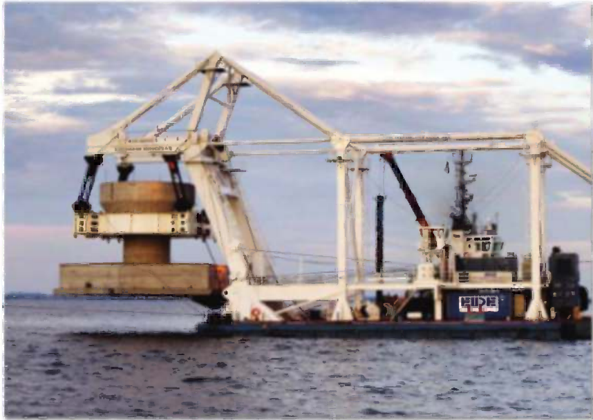
Lillgrund Wind Power Plant 2008-09-21 The foundations will be lifted up from the barge at Lillgrund
