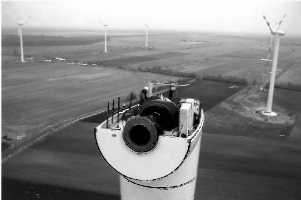
Figure 6.25 Turbine assembly in the air (1); View of nacelle of 1.5 MW NEG Micon turbine after installation of low-speed shaft (front) and gearbox. The ring of bolt holes in the low-speed shaft for hub mounting are clearly visible. Reproduced by permission of NEG Micon
