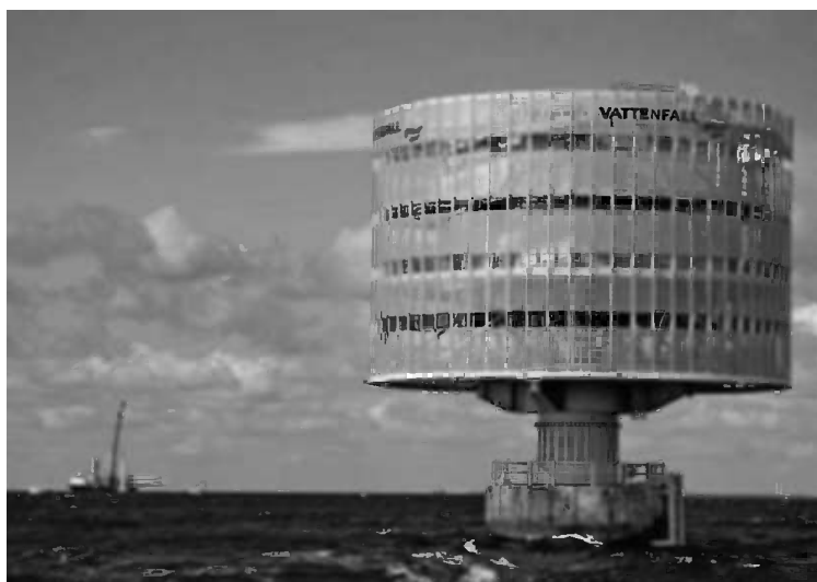
Figure 11.59 Offshore sub-station at Lillgrund. Lillgrund Pilot Project, 2008. Reproduced by permission of Vattenfall. See Plate 8 for the colour figure
