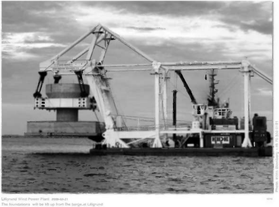
Figure 11.49 Lowering of gravity base by floating crane during installation at Lillgrund wind farm. (Lillgrund Pilot Project, 2008). Reproduced by permission of Vattenfall. See Plate 5 for the colour figure
