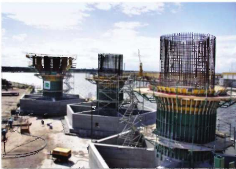
Lillgrund 2008/01/01 Windturbin foundation Swinoujskie Piering
