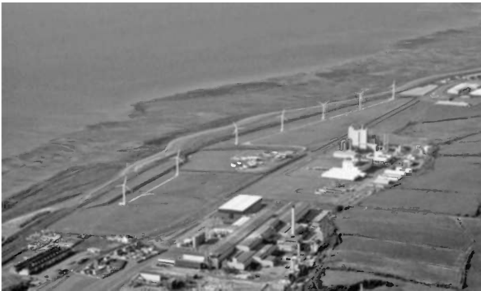
Figure 9.5 Wind farm of 700 kW wind turbines located along coast. Reproduced by permission of PowerGen Renewables/Wind Propsect Ltd.
