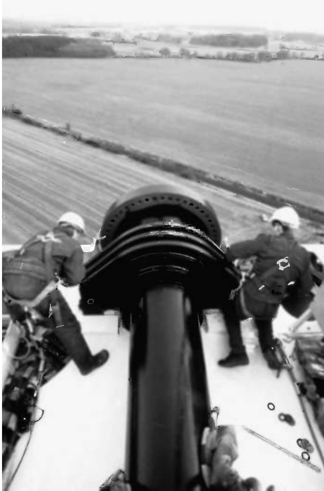
Figure 6.26 Turbine assembly in the air (2); View of low-speed shaft and front bearing after installation on 1.5 MW NEG Micon turbine. Reproduced by permission of NEG Micon
