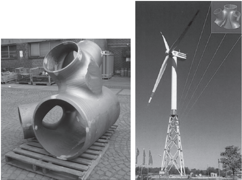
Figure 8: Prototype of a REpower 5M offshore wind turbine in Bremerhaven, Germany with casted joints [12, 13].
