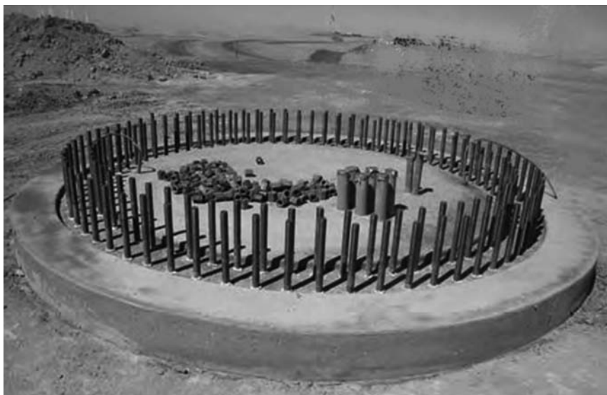
Figure 38: Tubular tower foundation after pour and backfill – tower ready [41].
