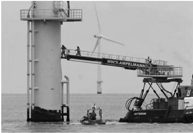
Figure 37: Ampelmann system for accessing offshore wind turbines.
