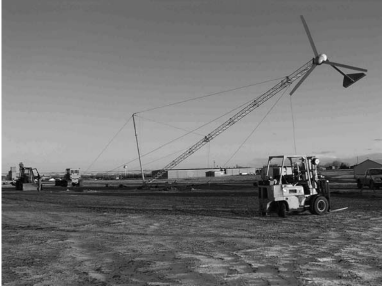
Figure 9: Bergey 10kW with tilt-up tower and furling tail (credit: AWEA, Don Marble).
