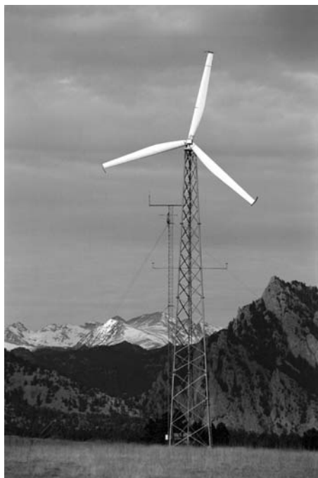
Figure 6: AOC 15/50 (credit: AWEA, David Parsons).
