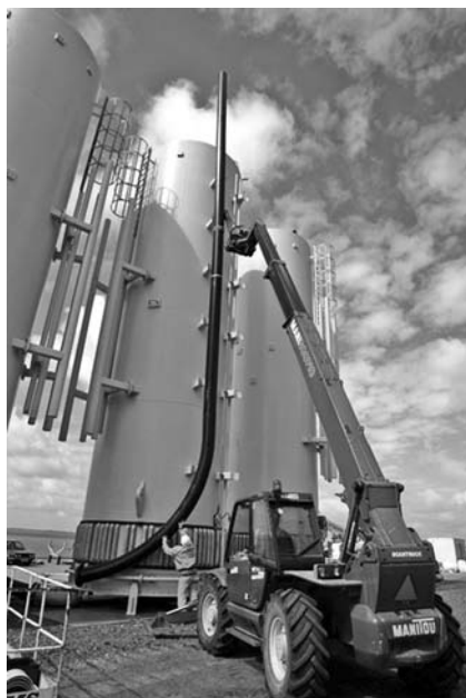
Figure 14: The J-tube through which the power cable is directed to the seabed.
