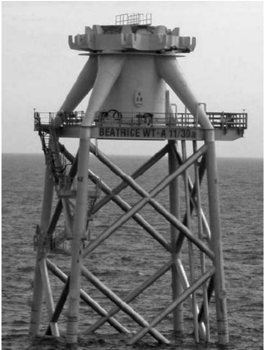
Figure 7: Repower 5M quadpod offshore foundation installed in 2006 [12].
