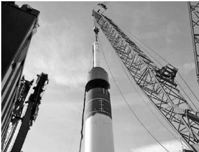
Figure 6: Pile hammering at Arklow [3].
