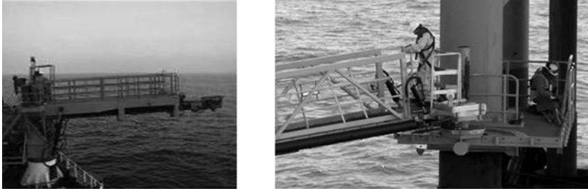
Figure 36: Access to offshore structure with OAS.
