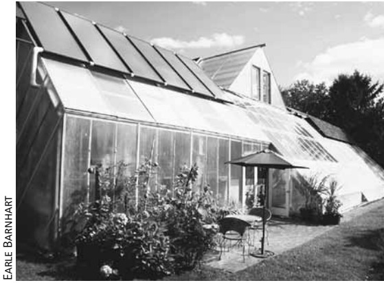
Ark 2010 South Wall Exterior
