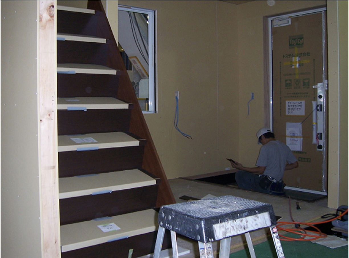
Figure 4.6 Offline module (customized stairs take a lot of labor that varies with choices).
