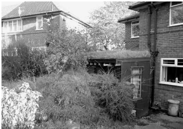
Green roofs needn't be large and expensive. This is a simple one on a garden shed.
