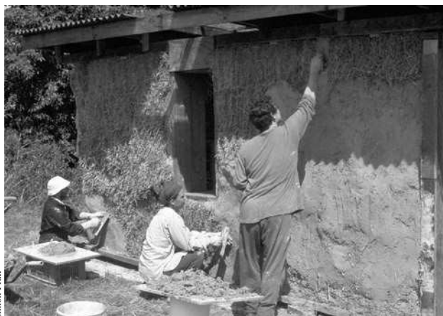
Putting the render on the walls of a straw bale building.
