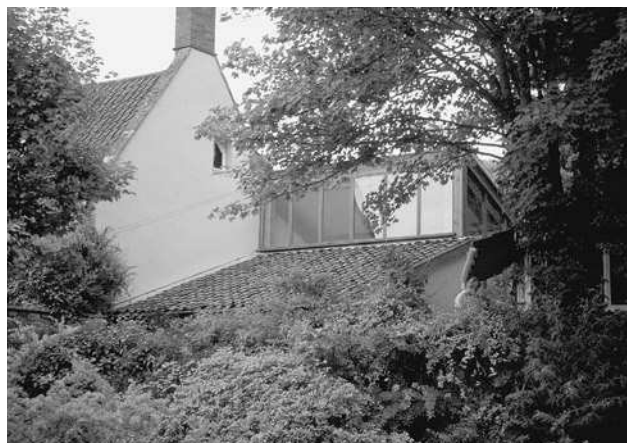
This recent extension has been given a clerestory window to give full natural lighting to its single large room.
