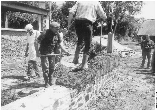
A new cob wall goes up on a foundation of stone.
