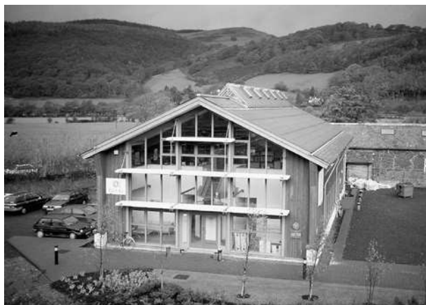
Passive solar heating can be specially effective in commercial buildings because they're occupied mainly during daylight hours, which means heat can be used directly and heat storage is less important, as in this building on a rural industrial estate at Machynlleth, Powys.
