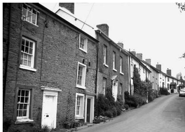
Terraced houses can be pleasant places to live, and they're much more energy efficient than detached houses.
