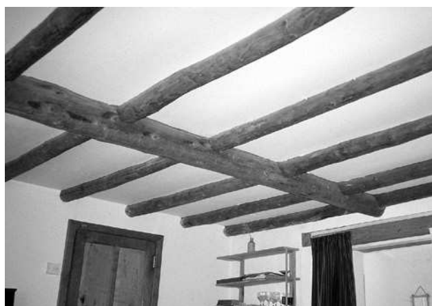
In this traditional Welsh longhouse roundwood has been used in renovation, providing the joists for a new ceiling.
