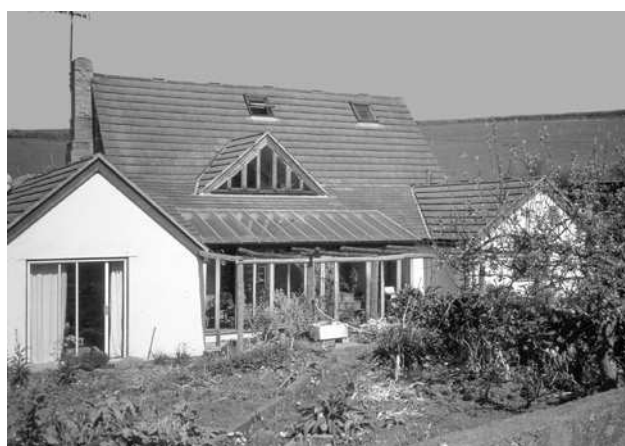
Winter, night-time. The conservatory heats the house by radiant heat.
