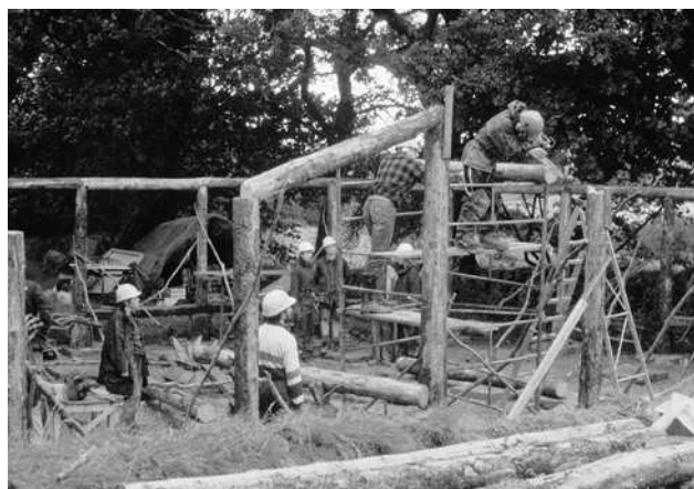
Roundwood frame for a dwelling house under construction at Brithdir Mawr, Pembrokeshire.
