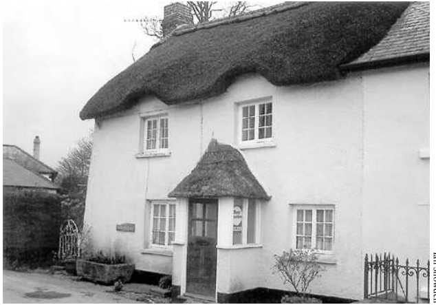
Only the tapering wall gives a clue that this cottage is built of cob rather than a more conventional material.
