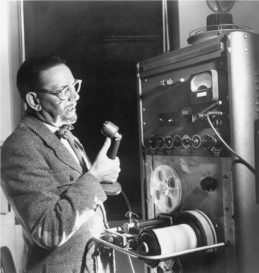
Bell Telephone Laboratories engineer Lawrence G. Kersta invented the sound spectrograph, a machine that turns spoken words or other sounds into visible tracings. Some forensic analysts use the sound spectrograph to identify individual voices. (Lucent Technologies Inc.)
