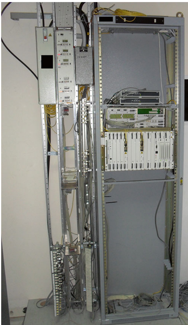
Fig. 3.2 Large size office demarcation point
