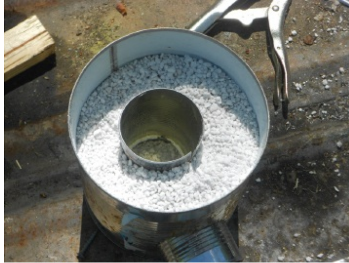
Figure 41.12 Fill with insulation.
