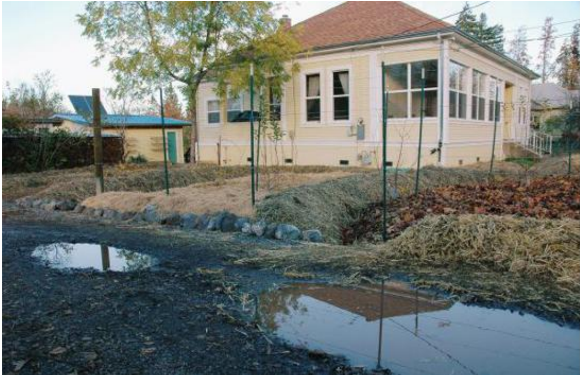
Newly installed earthworks including swales, berms, permeable pathways, French drains, and keyhole planting in this Willits, California yard. The standing water seen in the foreground was common throughout the site before the earthworks, compost, and mulch were installed. Posts for trellising the mini-food forest can be seen where the lawn once was. In the background is the downspout leading to the water storage under the house and to the left the garage/guest room features trellises for vertical gardens in front of it. Design by Maximillian Meyers of the Mendocino Ecological Learning Center. PHOTO BY MAXIMILLIAN MEYERS.
