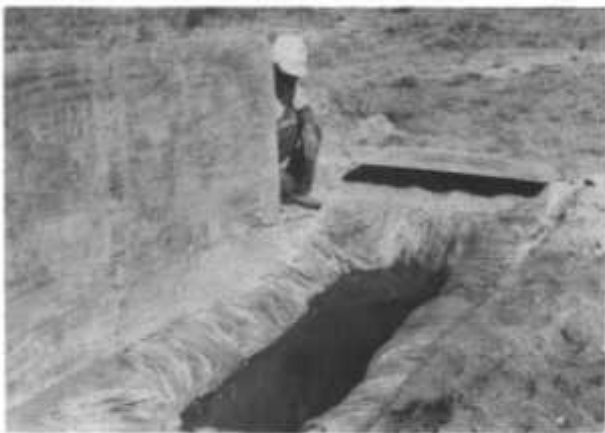
Fig. 8.5. View of plastic-lined water storage pit. This pit held about 200 gallons.
